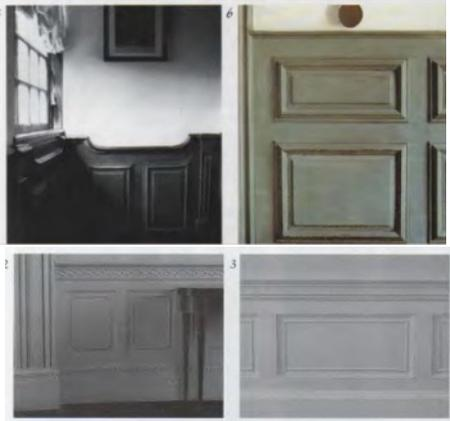
**Gambar 3. 2** Moulding Pada Dinding
