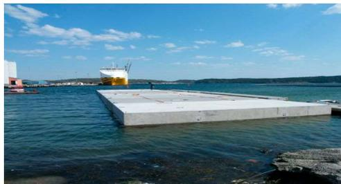
**Gambar 2. Fondasi ponton (Sumber : b-foam, 2015)**
